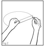
1. Determine the position in ceiling 2. Use the template provided where fanlight is required to be to draw a circle 300mm in diameter. To do this insert a 120cm of stove or inside a shower thumb tack in hole at one end and insert a pencil in the other installation area is not restricted hole and scribe a circle. refer table for clearance required
